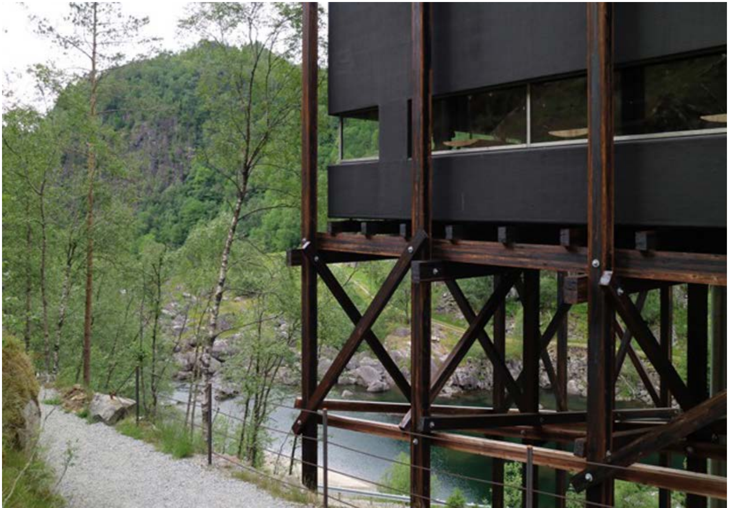
exposed structural framework on the prefabricated building image © atelier peter zumthor & partner
